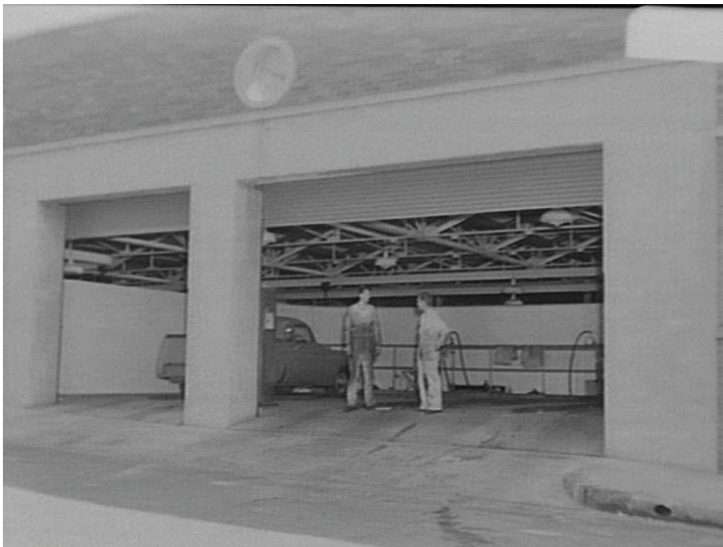
Figure 2.30 The Greasing Bay of the 1947 extension; this facility was accessible from Wentworth Street. Photograph is dated 1953
