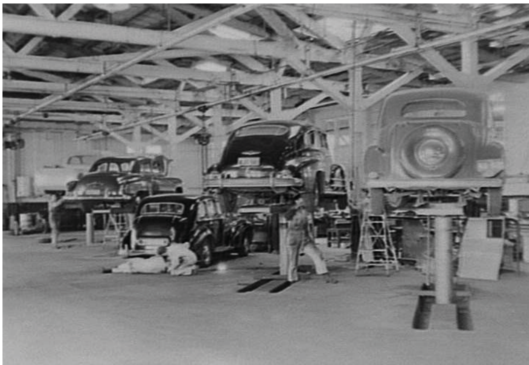
Figure 2.19The hardwood structural frame of the 1913 garage. Photograph is dated October 1953
