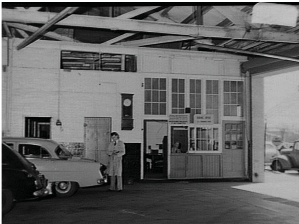
Figure 2.20 The administrative offices of 1913 building, which were located to the east of the two-storey section. Photograph is dated October 1953
