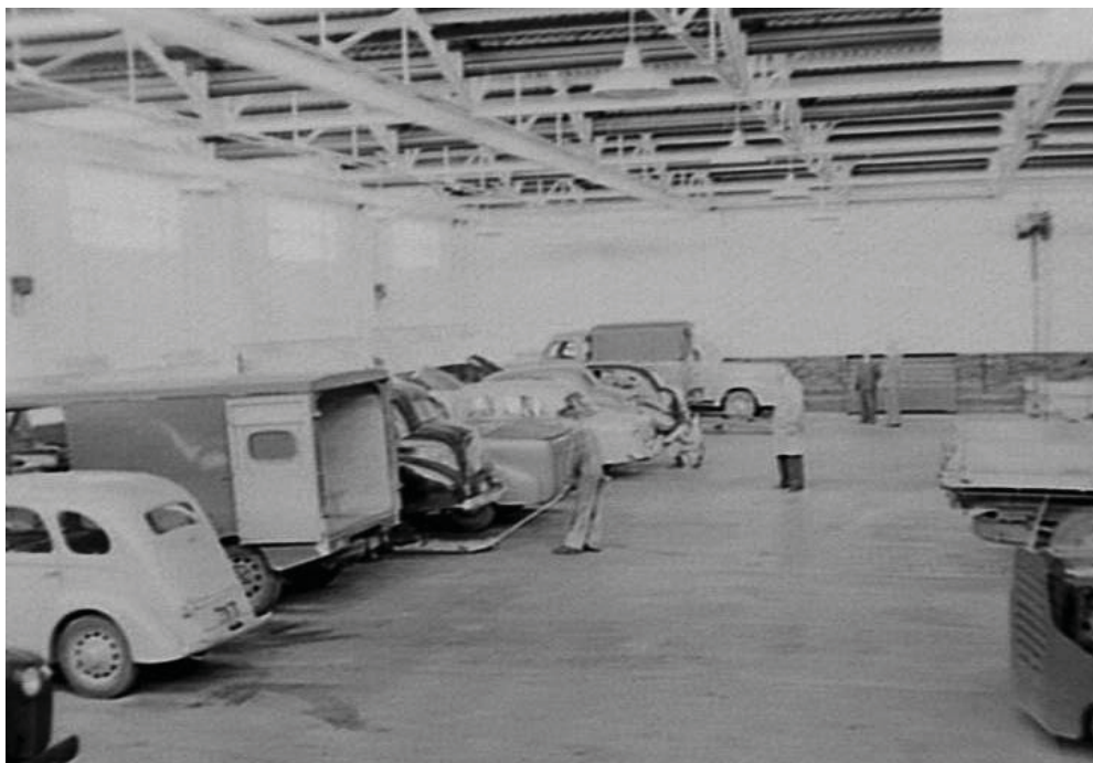
Figure 2.31 The servicing area of the 1947 garage extension
