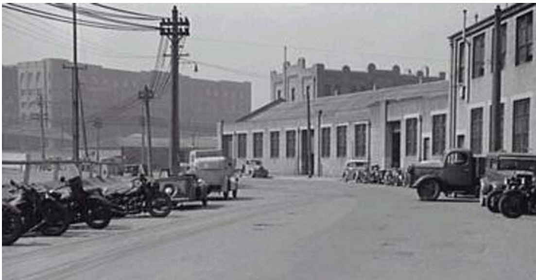
Figure 2.15 The Wentworth Park Road frontage of the State Motor Garage. The photograph shows alterations to the openings of the western section of the garage. Undated, 1930s
