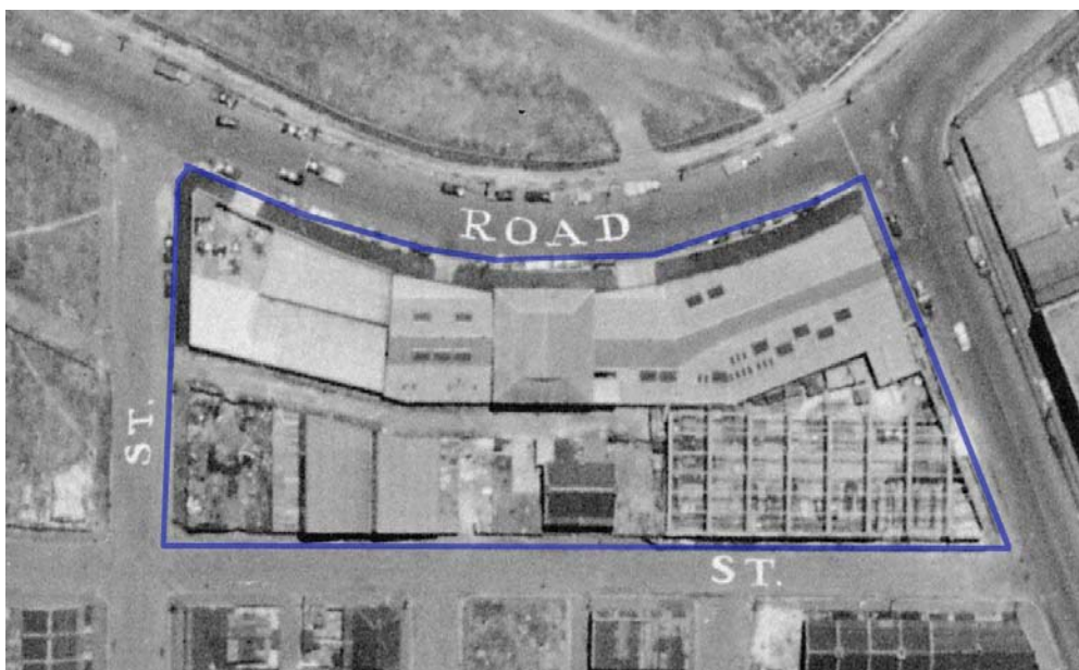
Figure 2.24 The site in 1949. The photograph shows the garage extension along Wentworth Street under construction and the site of the old stables in Wentworth Park Road redeveloped
